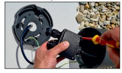
6. Feed the power supply cable through the cable gland.
